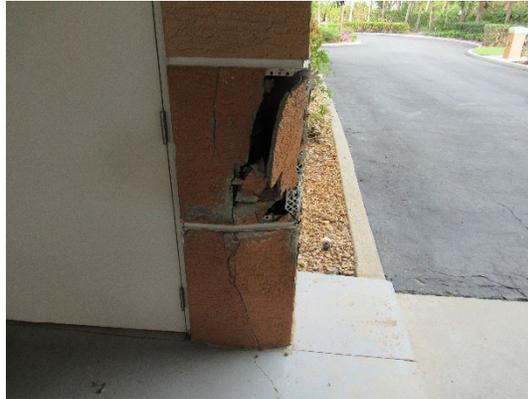
A photograph showing a brick pillar in a garage. A large, jagged hole has been made in the brick and stucco, with a car's bumper visible at the top of the opening.                       |
