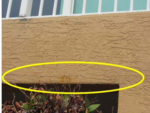
A photograph of a textured, light-colored stucco wall. A yellow oval highlights a horizontal crack in the stucco, with a yellowish-brown stain below it, indicating corrosive staining. |
