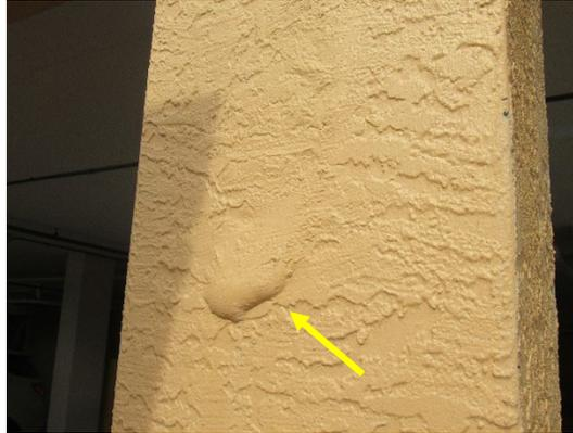
A close-up photograph of a textured, light-colored stucco wall. A yellow arrow points to a small, raised, circular area on the surface, which is a typical paint blister.                |
