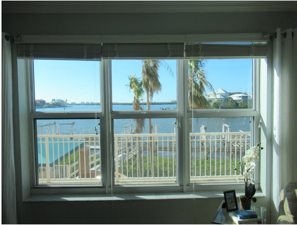
Overview of a window in unit 107.
