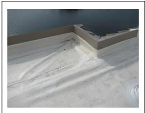
View of unadhered roof membrane and bent flashing.
