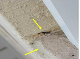
View of hole in the stucco and delaminated concrete on the 4<sup>th</sup> floor breezeway.
