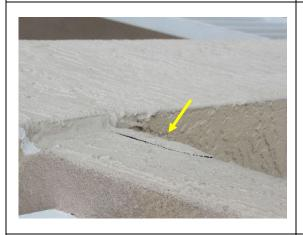
View of delaminated stucco on the PH floor breezeway.
