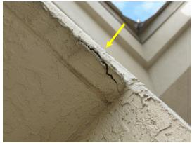
View of delaminated stucco on the 6<sup>th</sup> floor breezeway.
